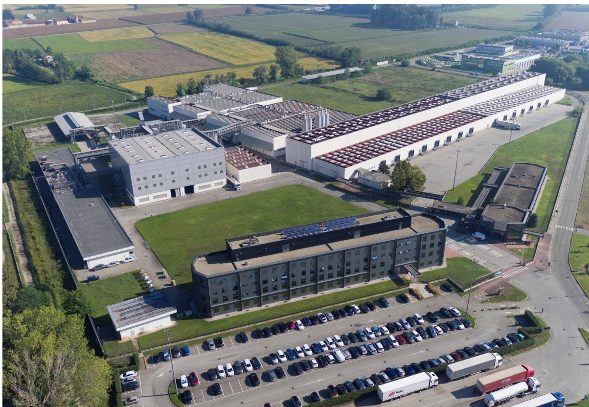
Figure 2. IVM Chemicals Parona integrated resin and paint production site
